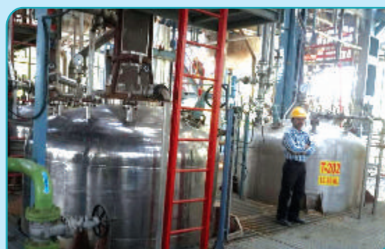
India's first 2G or cellulosic ethanol demonstration plant with a capacity of 10 t/day erected at India Glycols Ltd., Kashipur
