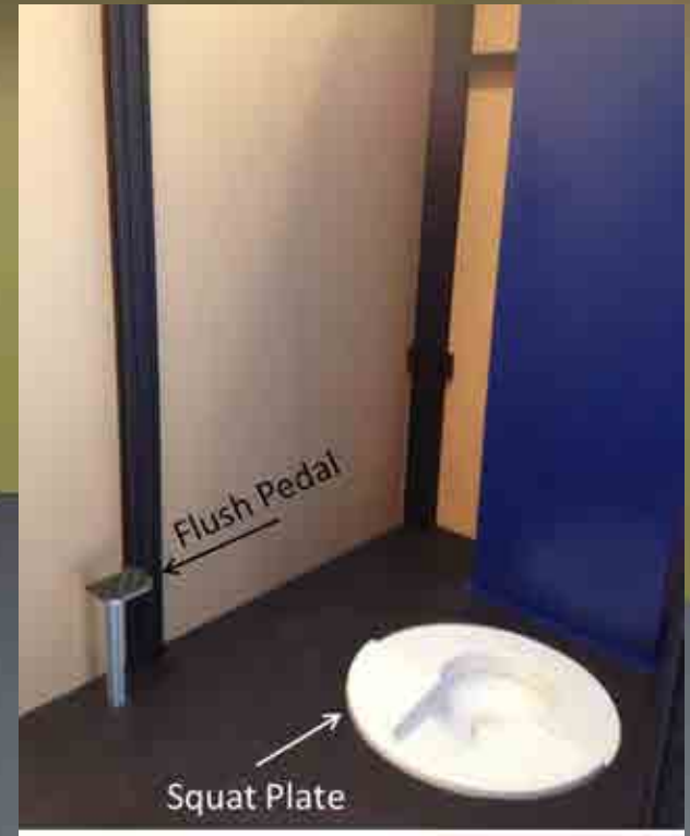
Custom RTT squat plate (Roca) (1.5 L per flush)
