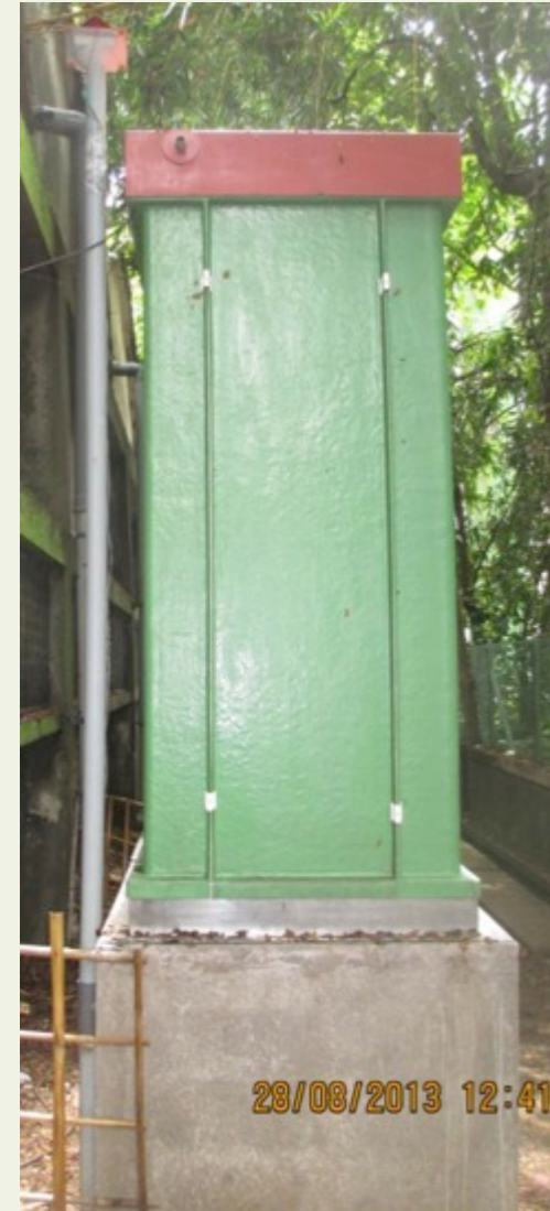
Vent pipe for solids pit
