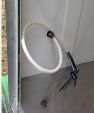
Jet spray for anal cleansing
