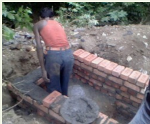
Pits under construction
